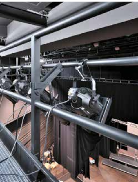
Passerelle de face, lisses basculantes (MHS17)
