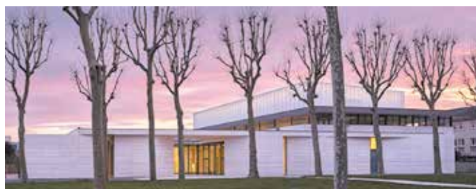
Rambouillet, facade - Photo © Studio-Milou
